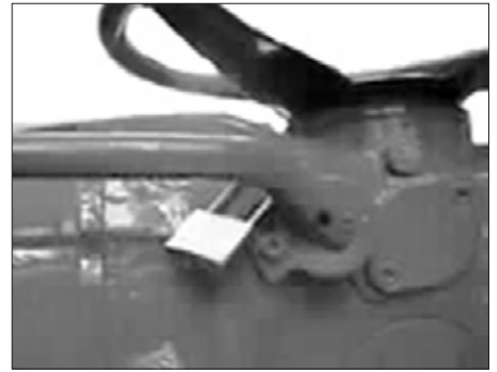
Engagement lever locked in motor operation position: the manual operation cannot be engaged, and this excludes unwanted local operations.
