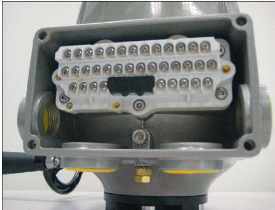
FIGURE 13 - Overview of the cable entries conduits.
