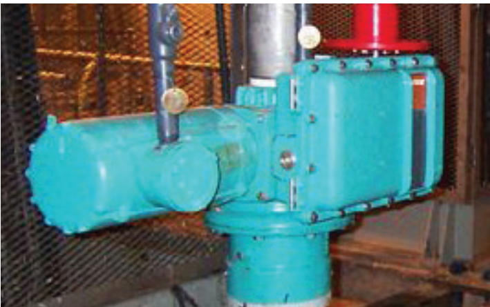
Bettis AquaNaught variant of the M2CP actuators can withstand extended submersion.
