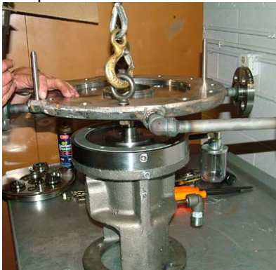
Seal housing being installed onto bearing box.
