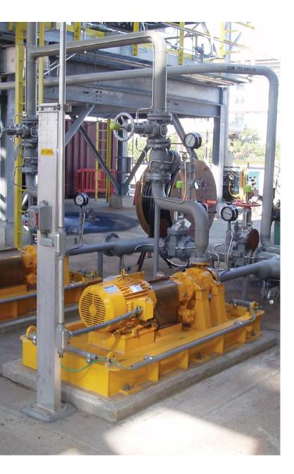
The GSP range comprises of pumps based on the HMD Kontro GS drive, built to API 685 specification, suitable for heavy-duty applications.
