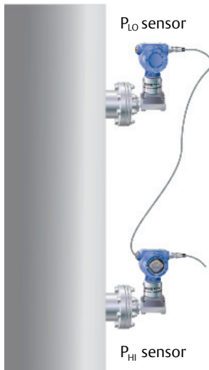
Figure 1. Vertical Rosemount 3051S ERS Installation
